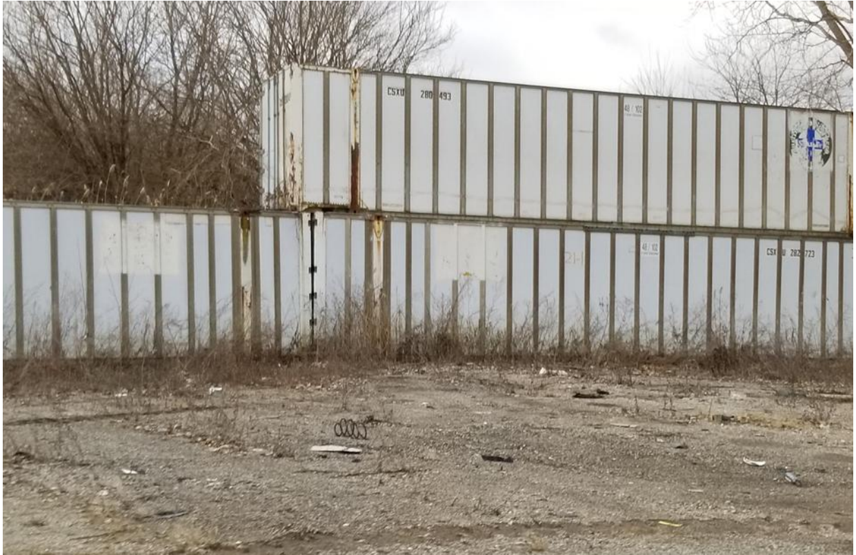
Shipping containers act as a perimeter barrier at Doty. Source: OIG photo
