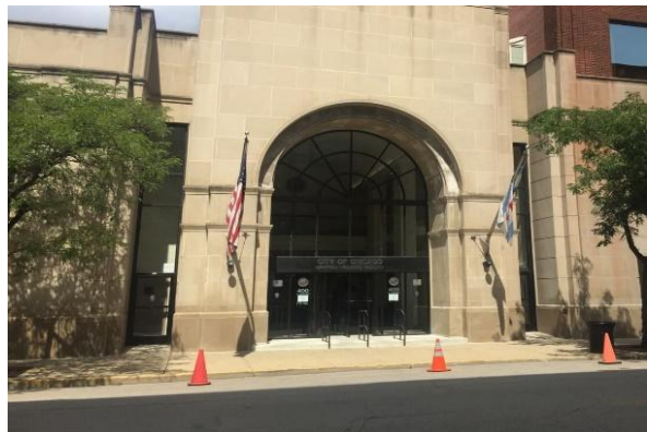
The City's Central Hearing Facility is located at 400 W. Superior St. Source: Public Building Commission, https://pbcchicago.com/projects/400-w-superior-building/ .
