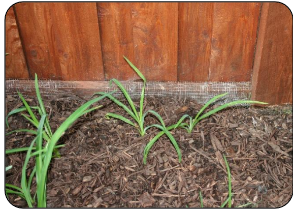
Wire mesh is used along a fence to prevent rats from entering a private yard. Source: OIG photo
