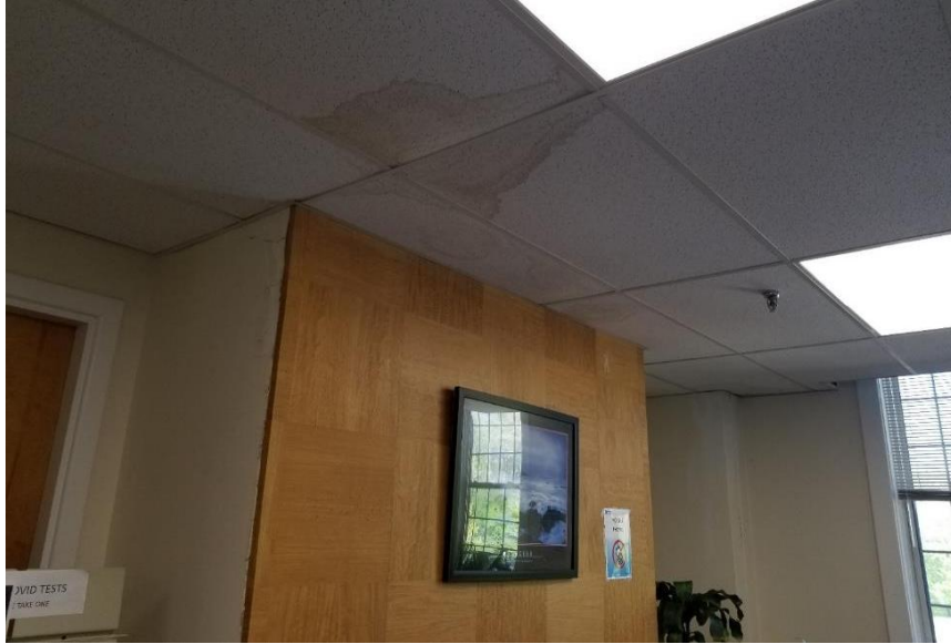
Water damage is evident in ceiling tiles at the North River Mental Health Center's waiting area. There did not appear to be an active leak at the time of OIG's visit. Source: OIG photo.
